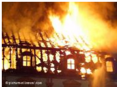
Fire caused extensive damage to Erfurt's Anna Amalia
